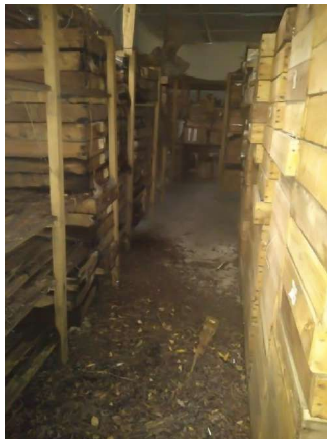
Figure 11: Inside the Archaeological Storage Room. Notice rainwater-drenched surface in the storage room. This endangers the organic material collection. Revamp the roof and separate camping gear from the collection. Photo by George Ghandi.
