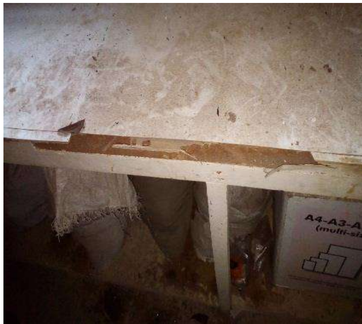
Figure 13: Inside the Archaeological Storage Room. Notice the action of termites and dust accumulation on the wall and fixtures. Regular cleaning and inspection is recommended. Photo by Maseno University attachment students of January-April 2021.
