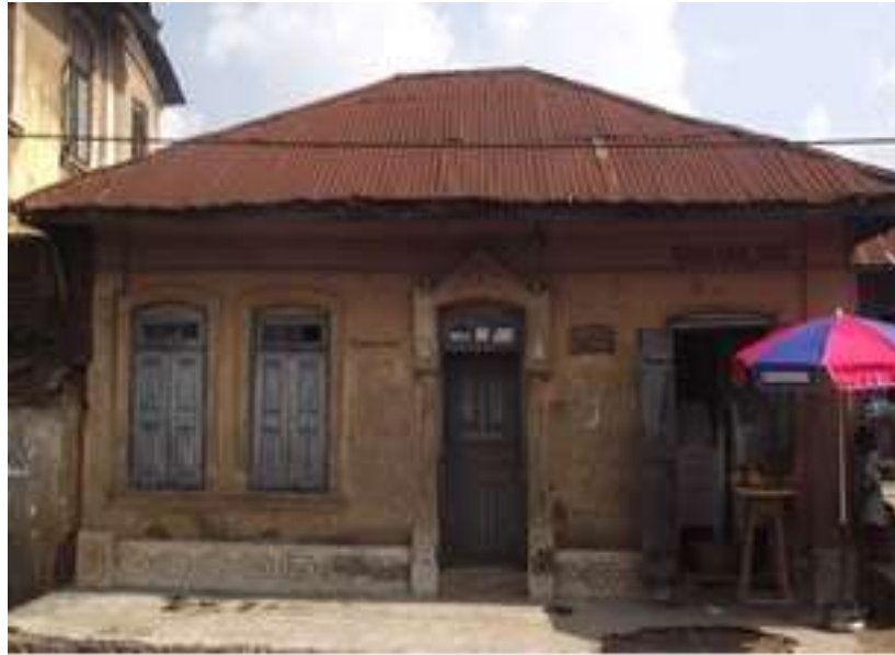
Plate 8c: A low-class bungalow at Ikija showing wall relief, dado and portals. Photography by: Kehinde Adepegba (2013)
