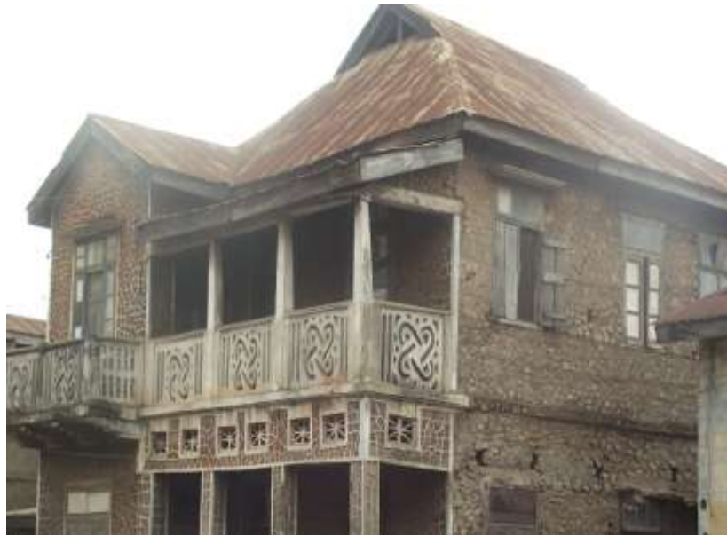
Plate 11c: House with repeated unity symbol (isokan) motif on the parapets..Photography by: Kehinde Adepegba (2013)
