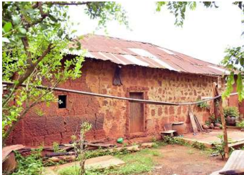
Plate 3, Traditional Yoruba buildings. Showing mud, woods, corrugated iron sheets and laterite.
