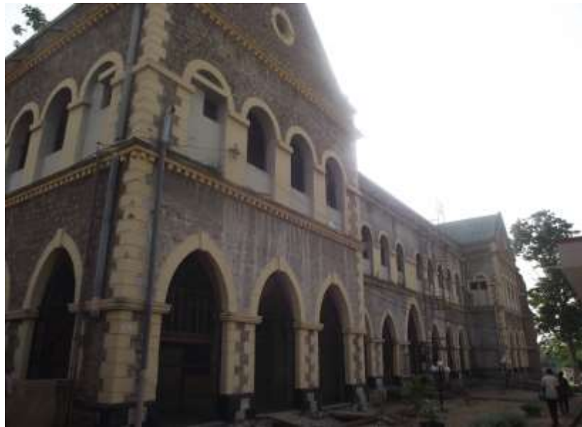
Plate 6a: Abeokuta Grammar School built in 1910. It was later used for subsequent takeoffs venue for Federal College of Education and University of Agriculture Abeokuta at different time. Photography by: Kehinde Adepegba (2013)
