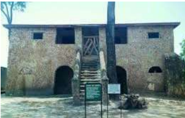
Plate 8: Surface corrosion, Colonial headquarters
