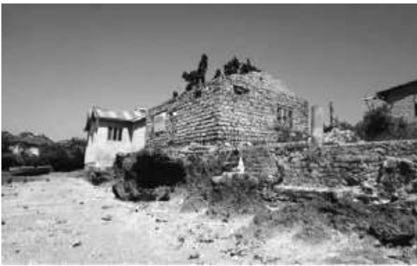
Plate 14: Eroded coral block building
