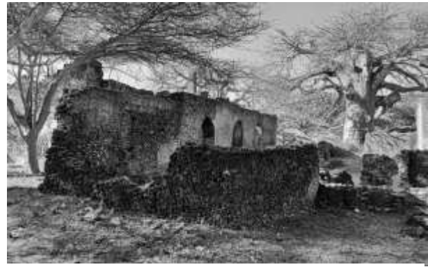
Plate 13: Eroded colonial armouries
